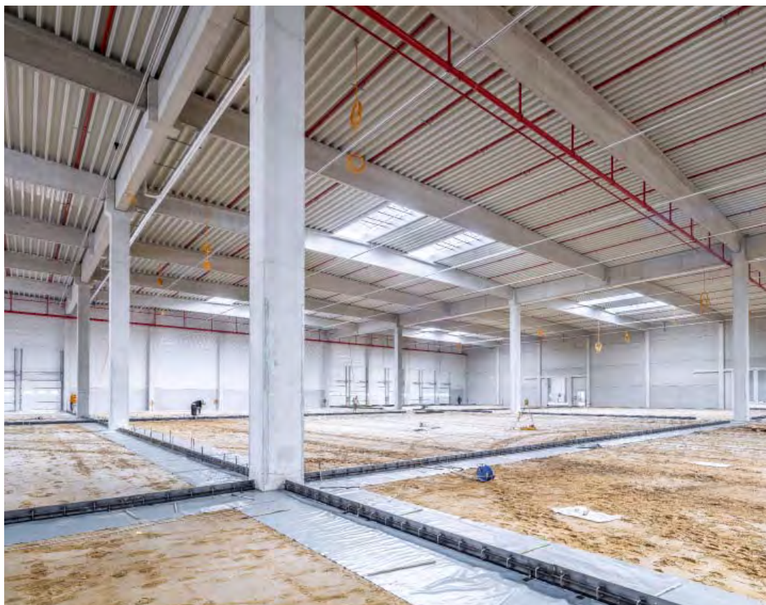
Works at VGP Park Soltau
