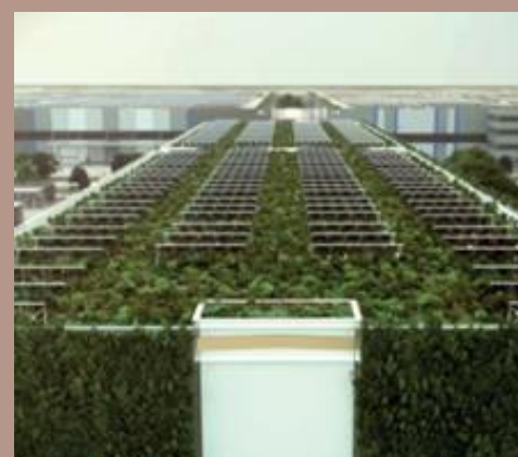
Green roof - Façade
