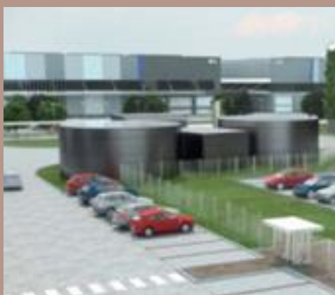
Groundwater heat pumps
